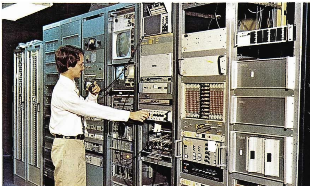
Tactec radio base unit in technical area at studio is used for expediting ENG microwave set-up.
